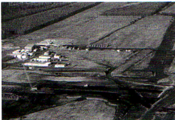
Fig. 7. Deep soil compaction by falling weight on future "Lusatian Ring" (aerial photo), BUL Sachsen GmbH.
