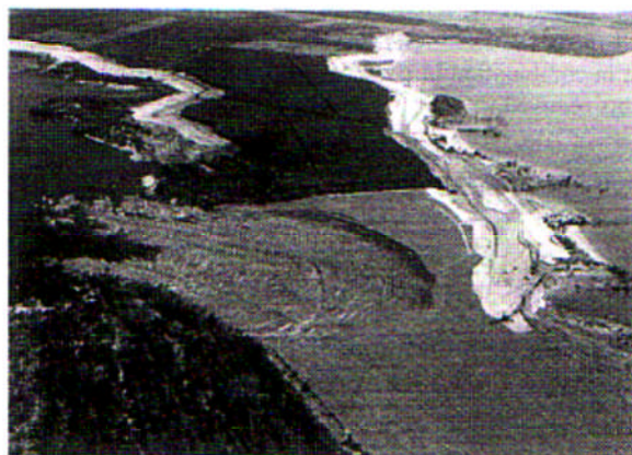
Fig. 1. Sliding, in 1998 (about 4.8 million m 3 ) on Koschen-dam near Senftenberg.
