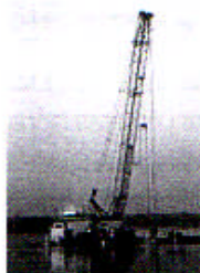
Figure 4: Compaction by vibration
