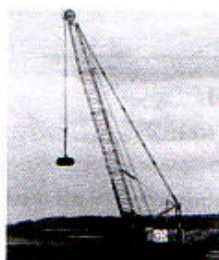
Figure 3: Compaction by falling plate
