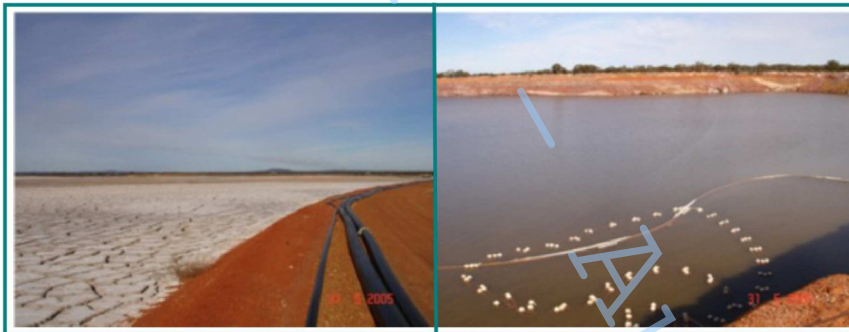
Fig.1 Gold mill tailings pond, WA (Goldfields)/Kalgoorly/hot arid climate zone/ left: free pond water infiltrated and evaporated; right: tailings pond with pond water lamella, photos by M. Lersow, 2005
