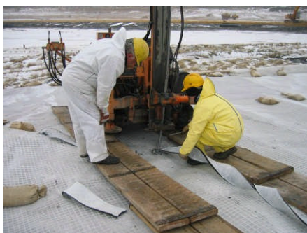
Figure 2 Installation of vertical drains
