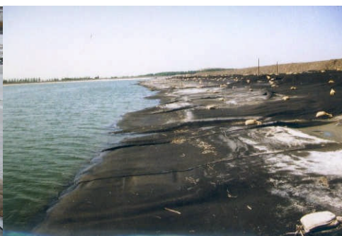
Figure 3 Stabilization of bank areas by means of sandmats
